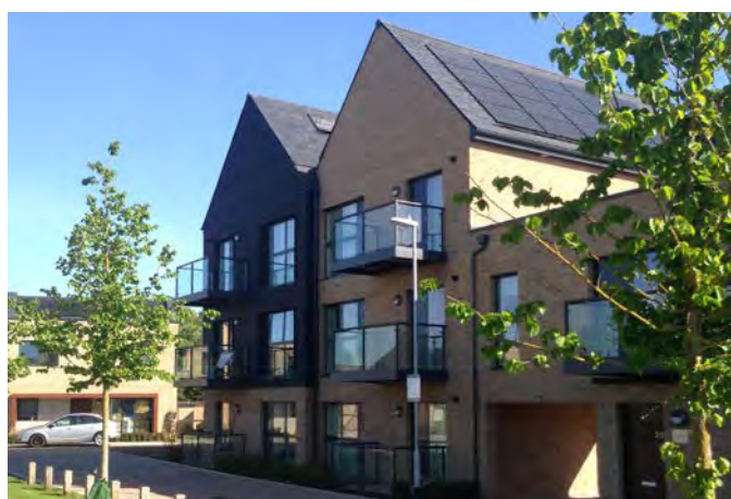
▲ The front and back of the home is clearly defined by landscaping and a front door facing the street. Private balconies are also provided for the homes without gardens.
