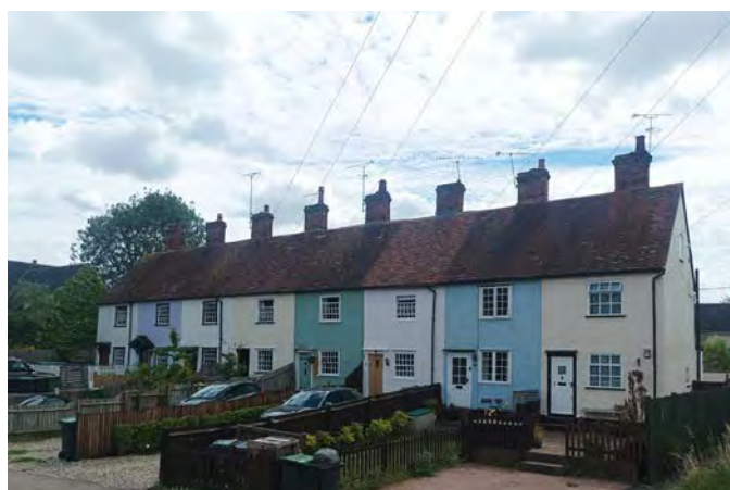
▲ Historic terraced homes come in a variety of colours and with a strong roofline in Church End, Great Dunmow.
