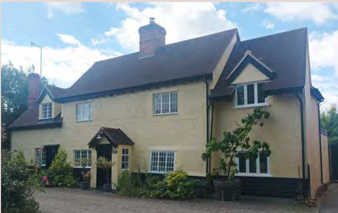
▲ Peg tiled roof, pargetting, dormer windows, central chimney and black weatherboarding on Dunmow Road, Takeley.
