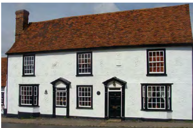
▲ The Bell in Great Easton, a former public house dating back to the 15th century, comprises of a timber framed building with plastered and pargeetting facades.
