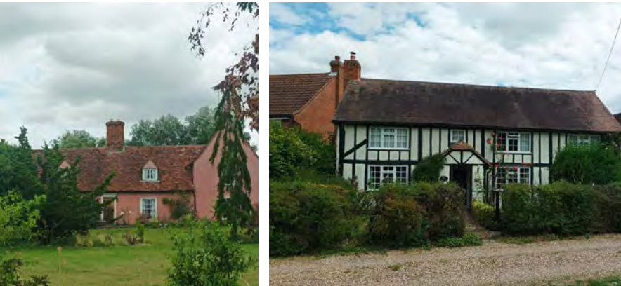
▲ Timber framed cottages with decorative facades in Free Roberts (left image) and Bannister Green (right image).
