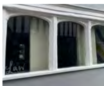
Wooden framed windows
